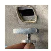
Hand tighten the Retainer Nut.
